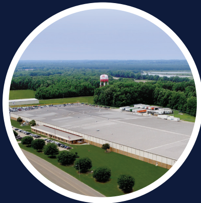
400,000 sq. ft. production, engineering, manufacturing facility
